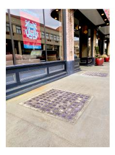
The ingenuity of replacing one large lens with smaller, thicker pieces of glass sustained the integrity of the sidewalk's safety. For building owners, vault lights added to property value and saved them considerable costs for electricity, which, at that time, was new and rather expensive. Hyatt became a successful and well-respected man, but his contributions to American history didn't stop at vault lights.
